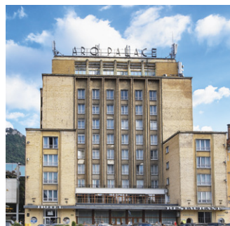
Aro Palace (1937-1938), arhitect Horia Creangă, Brașov – stil bauhaus
